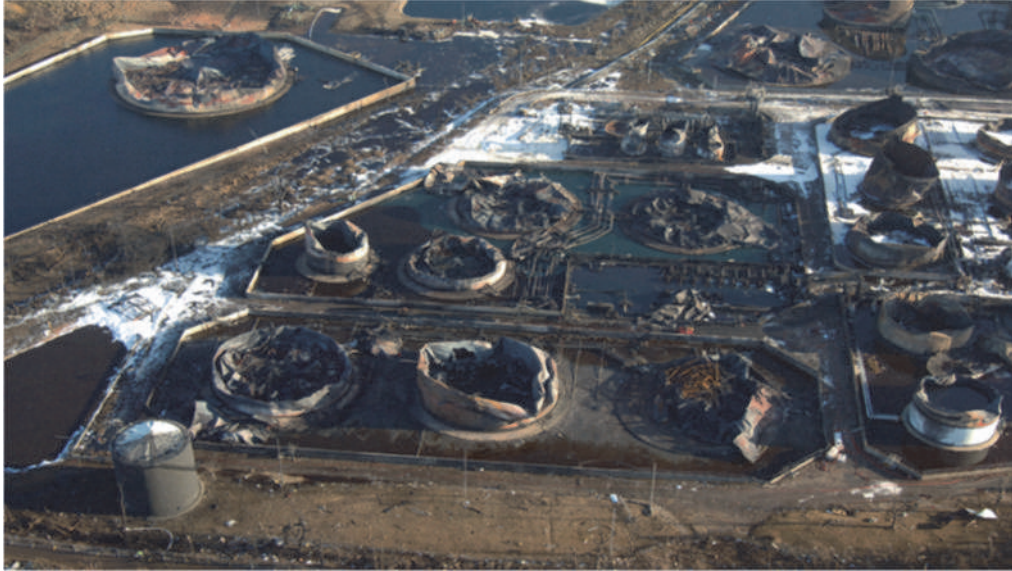
Figure 11.1. Buncefield storage depot after the explosion and fires (HSE 2011)
