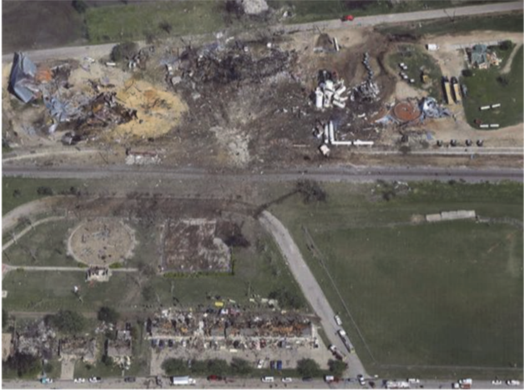
Figure 20.4. Overview of damaged WFC (CSB 2013)
