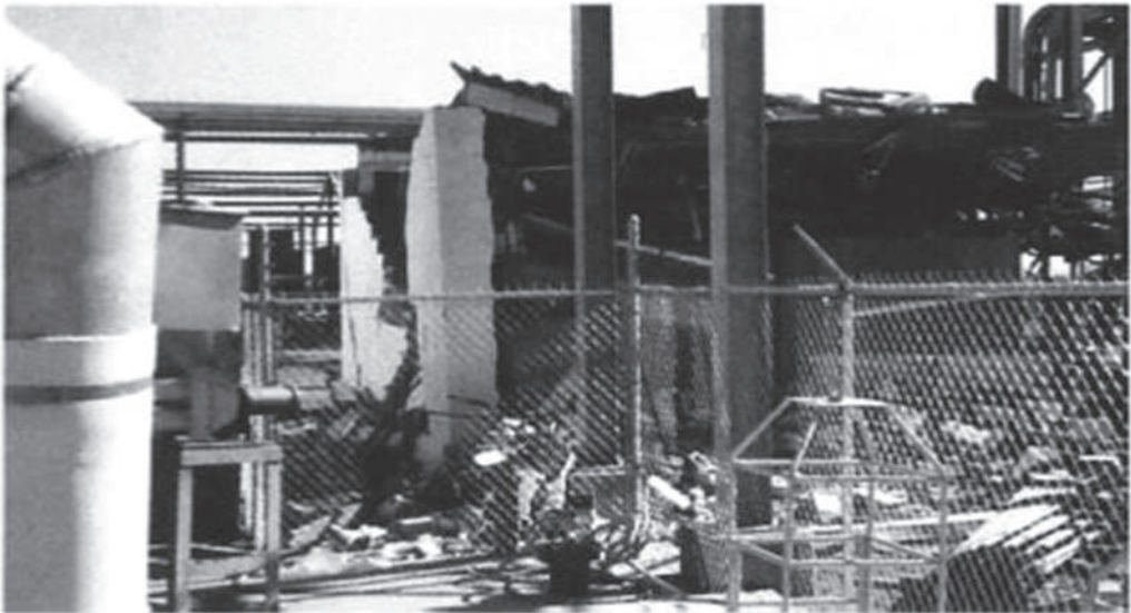
Figure 13.14. Pre-engineered metal building BDL3 (CCPS 2012) (Explosion Research Cooperative)
