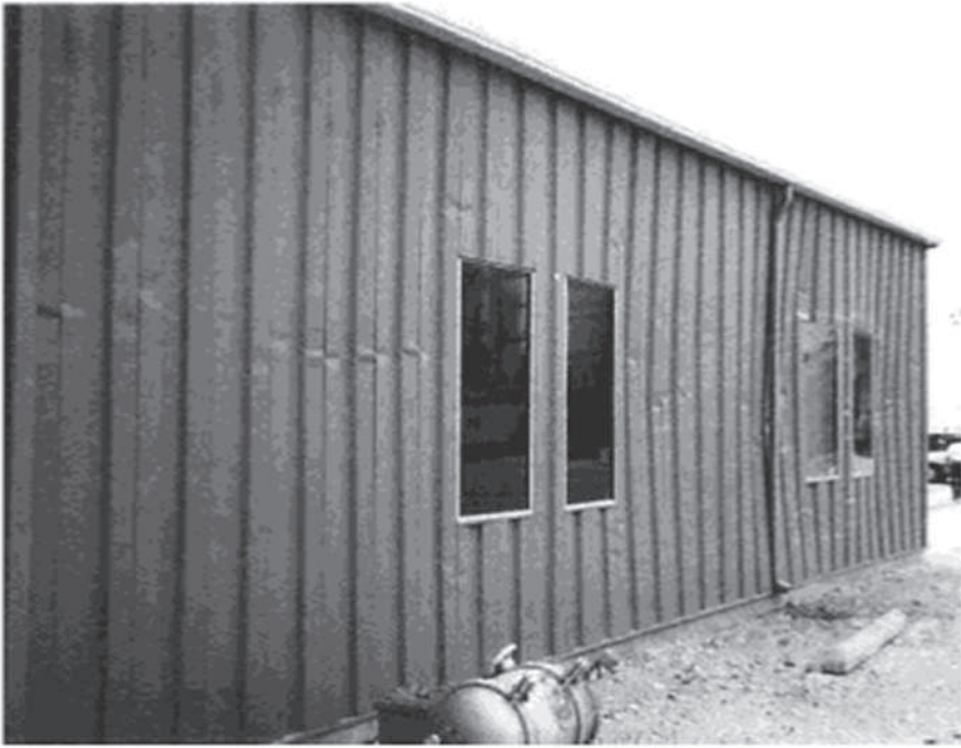
Figure 13.13. Pre-engineered metal building BDL1 (CCPS 2012) (Explosion Research Cooperative)
