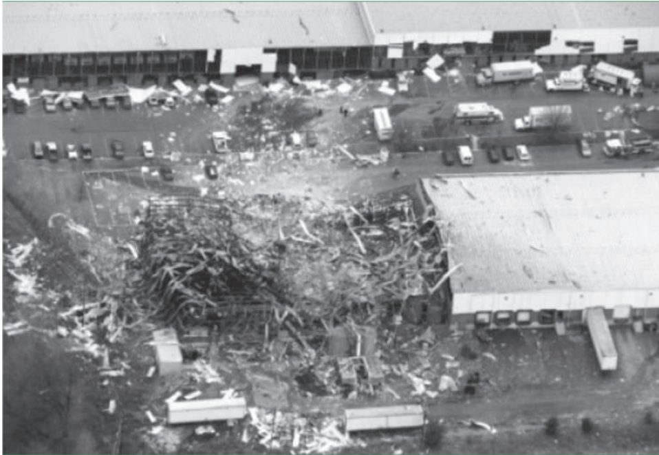
Figure 7.1. Damage to Concept Sciences Hanover facility Courtesy Tom Volk, The Morning Call (CSB 2002)
