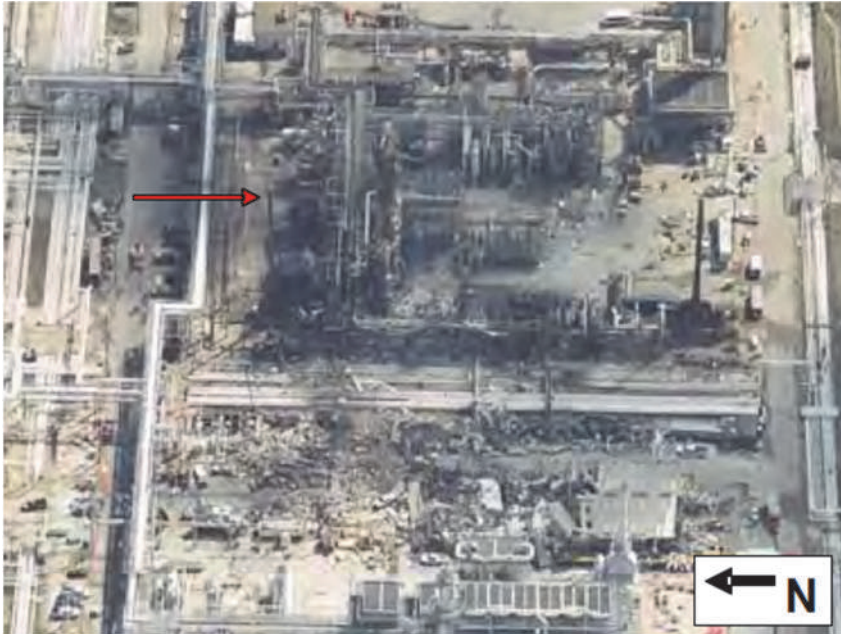
Figure 2.2. Texas City isomerization unit aftermath (CSB 2007)
