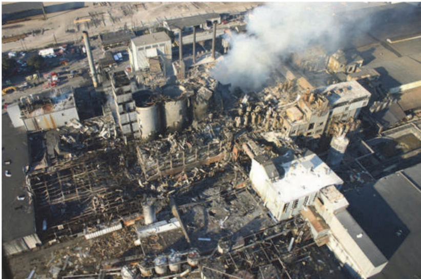
Figure 4.1. Imperial Sugar refinery after the explosion (CSB 2009)
