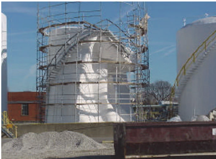
Figure 11.31. Tank collapsed by vacuum (CCPS g)
