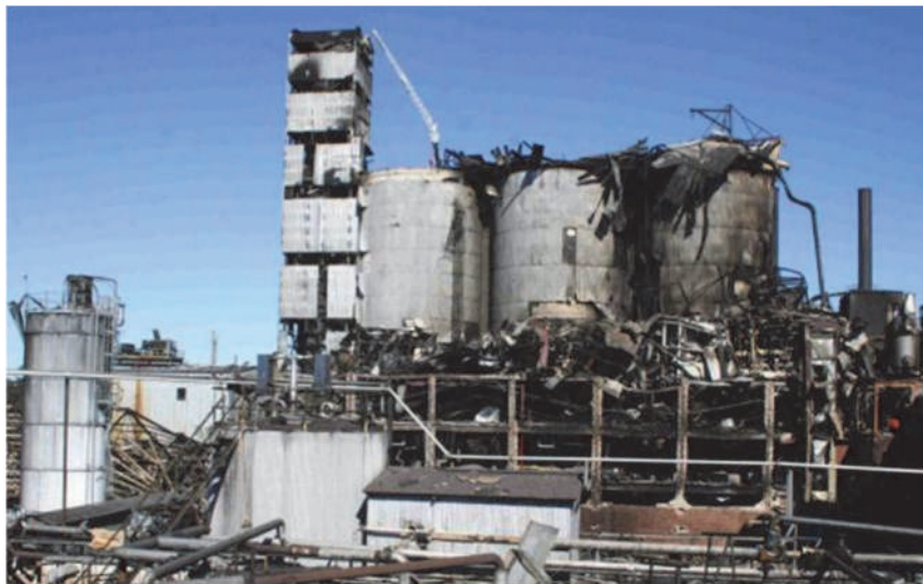
Figure 4.3. Imperial Sugar Refinery after the explosion (CSB 2009)
