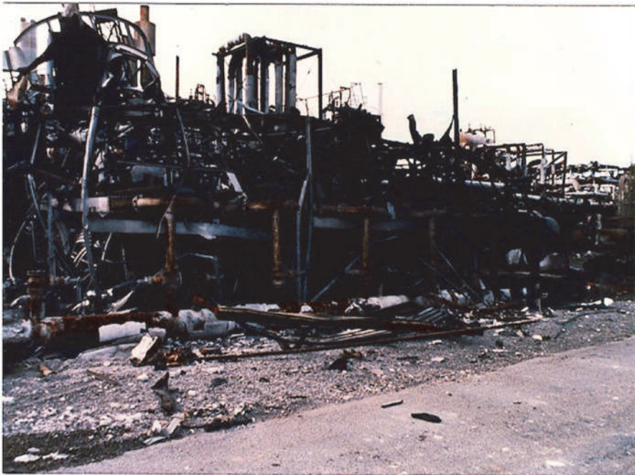
Figure 15.2. One of several units impacted by explosion (Celanese)
