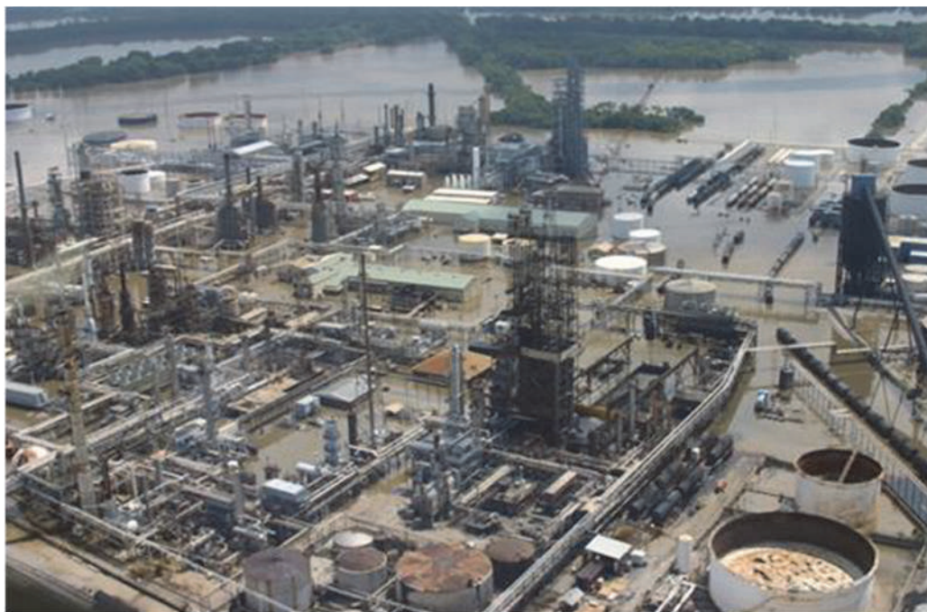
Figure 20.6. Coffeyville Refinery 2007 flood (KDA)
