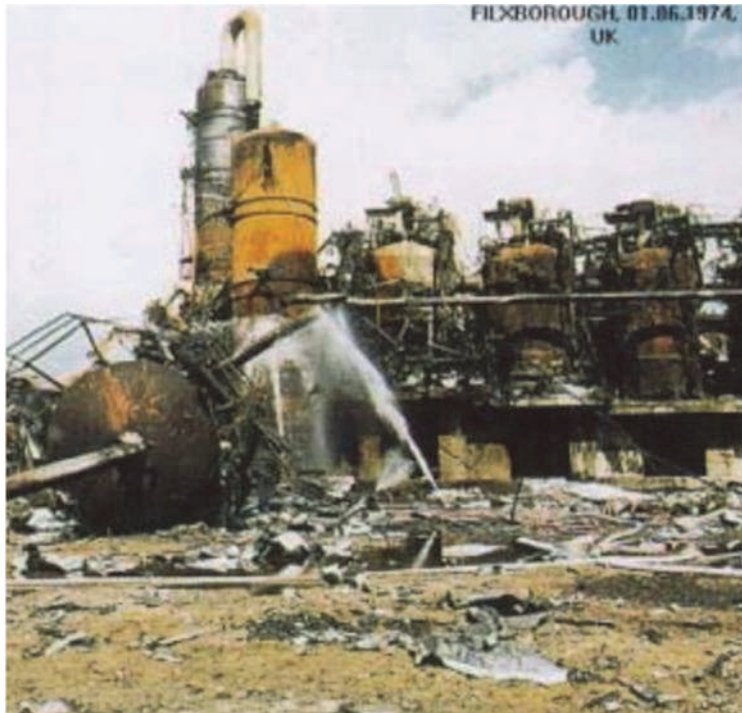
Figure 18.3. Flixborough site after explosion (CCPS 2005)
