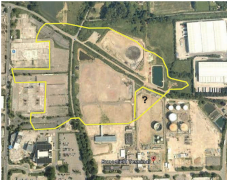
Figure 11.3. Buncefield Terminal site and wider area after explosion (HSE 2017)
