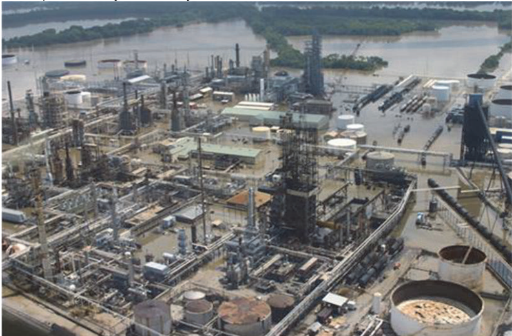
Figure 8.6. Coffeyville Refinery 2007 flood (KDA)
