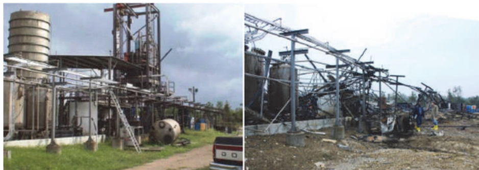
Figure 11.25. T2 Laboratories site before and after the explosion (CSB 2009)
